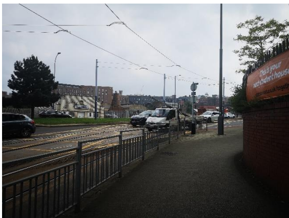
Yellow box junction in free flow traffic
