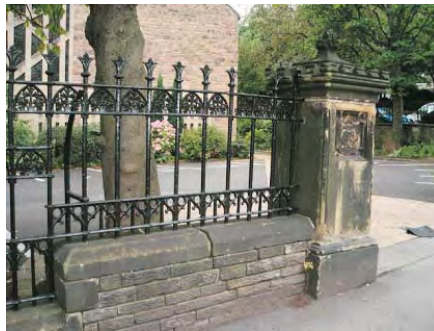
Railings beside St Mark's Church, Beech Hill Road
