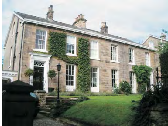
Nos. 13 and 15 Taptonville Road
