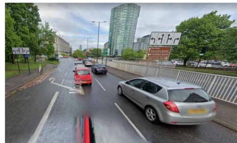
Approach to Moore Street Roundabout (image courtesy of Google Maps).
