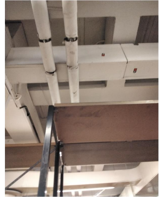
AIB to beams
