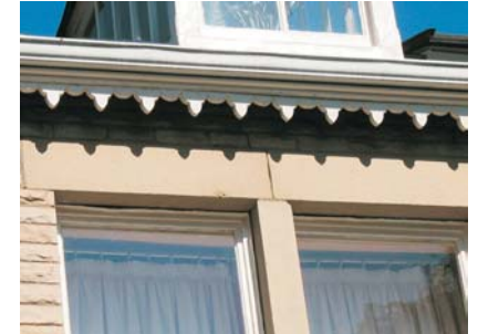
(l) Stone sills and lintels.
