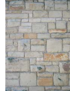
(q) Uncoursed squared rubble - common to side elevations and some inter war houses.
