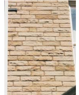
(r) Coursed stone typical to main elevations often in diminishing courses.
