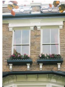
(i) Sliding sash windows constructed in timber.
