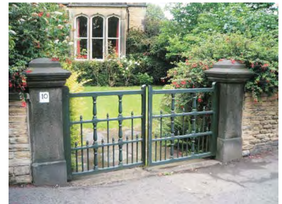
Gate to No. 10 Park Lane
