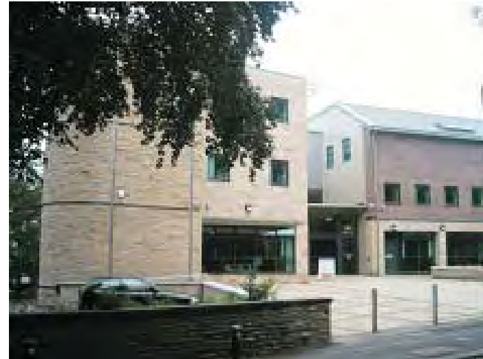
Modern Hallam University development, Broomhall Road building
