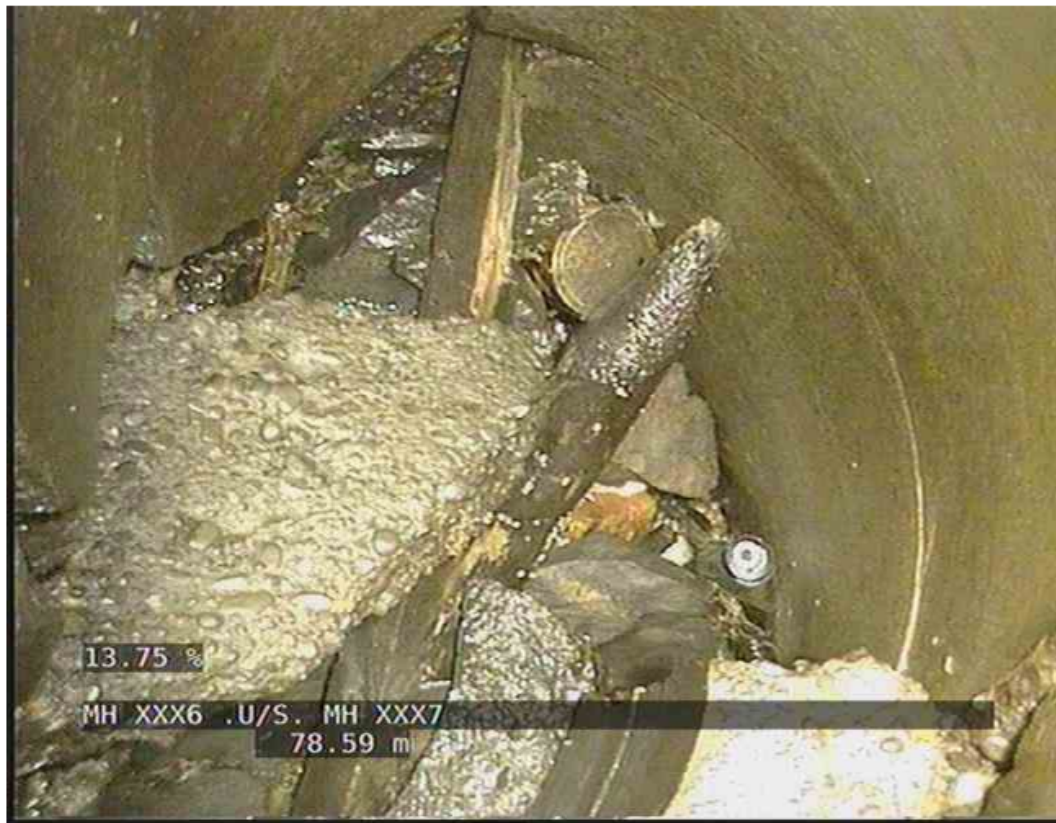
Figure 1: Image of failed and blocked culvert
